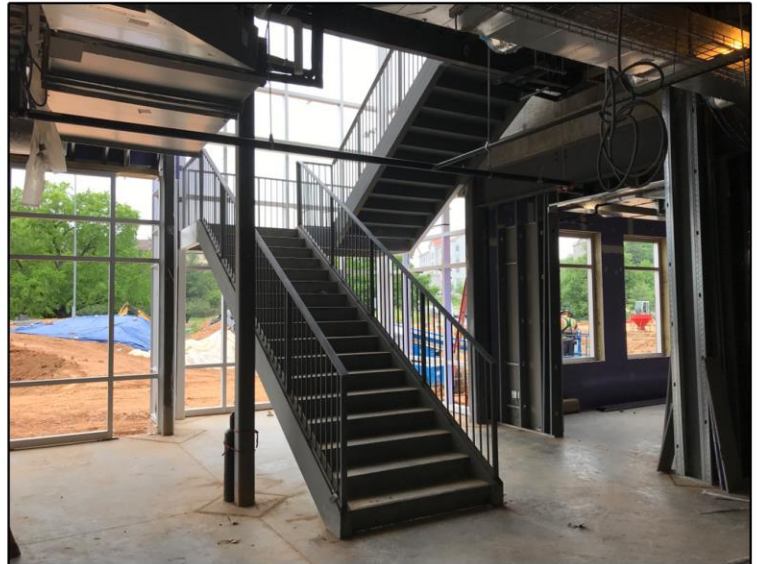
View of interior stairs leading up to the second floor
