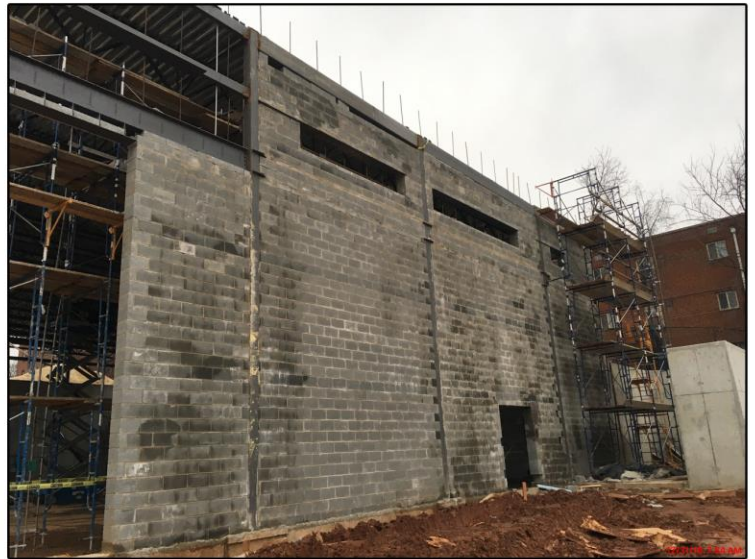
Construction team works to install concrete masonry units along south wall
