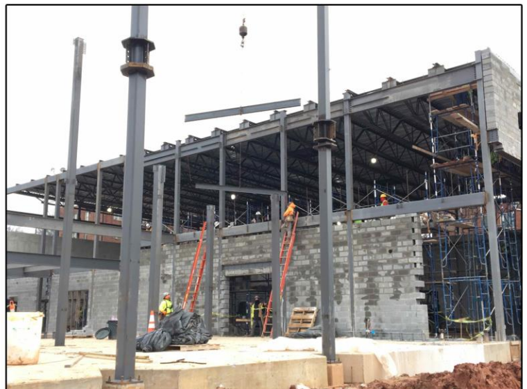
Construction team works to place remaining structural steel support beams
