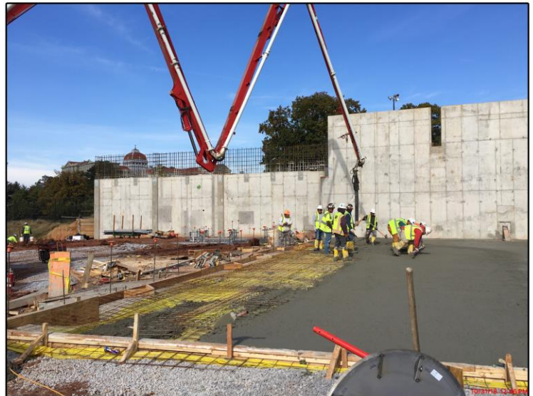
Construction team works to pour concrete slab on grade
