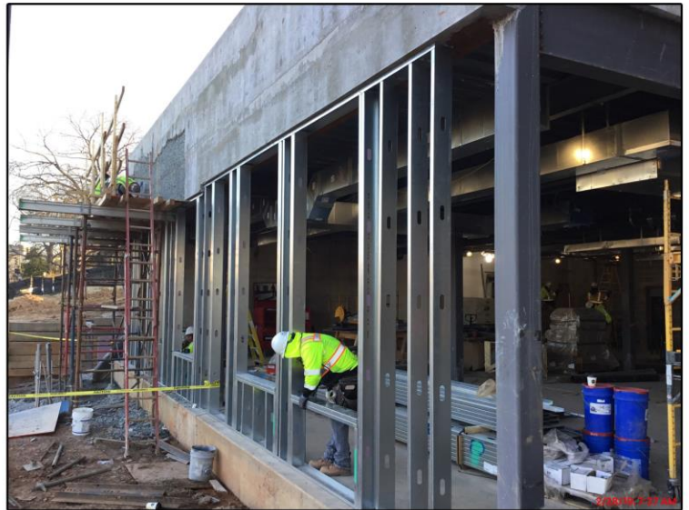
Construction team works to install exterior metal framing
