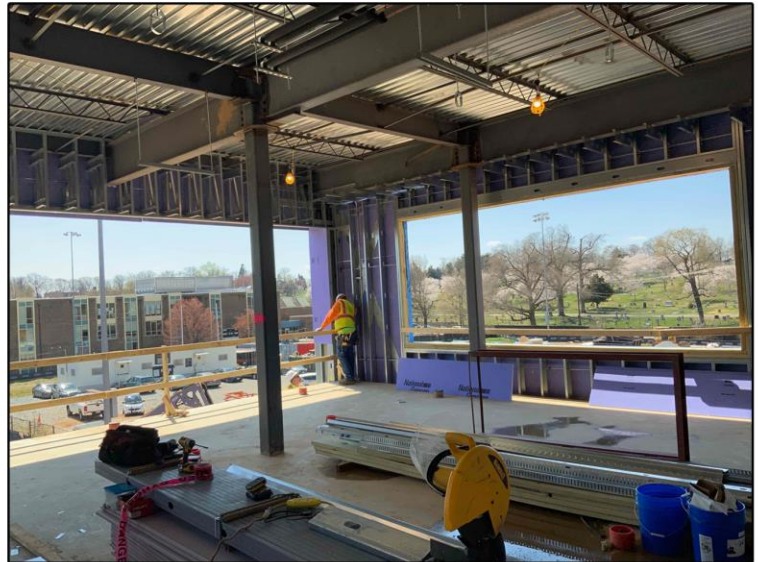
View from second floor fitness room towards Inspired Teaching School
