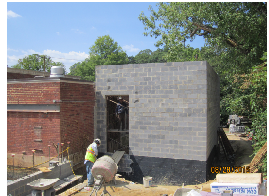
North Expansion CMU Walls
