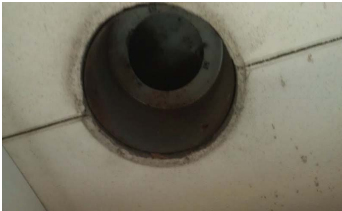
13. Assumed Asbestos-Containing Light Shields in Hallways. Not Sampled
