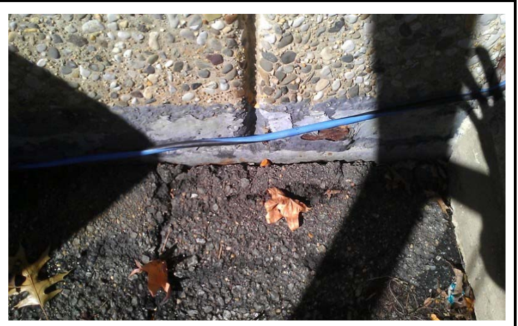
6. East Side of Building – View of Exterior Gray Waterproofing, Samples # E03-E04
