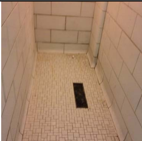
15. Assumed Asbestos-Containing Ceramic Floor Tile Mastic/Felt in the Bathrooms. Not Sampled.
