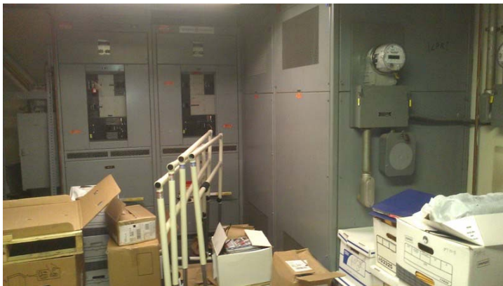
17. Assumed Asbestos-Containing Electric Panel Cement Components in Mechanical and Electrical Rooms. Not Sampled.
