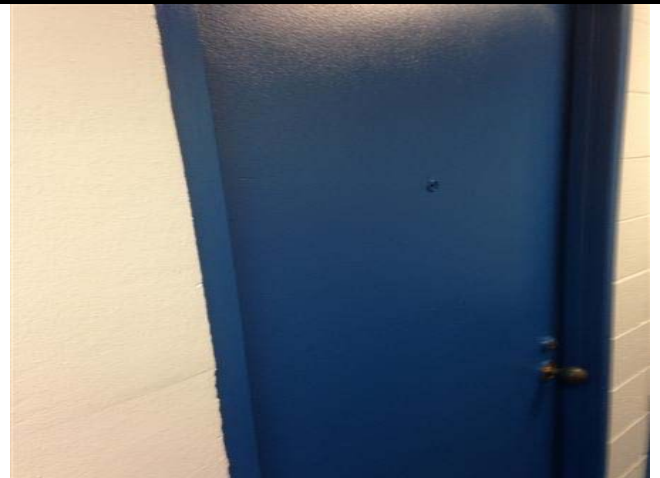
24. Lead-Based Paint on Blue Metal Window Door and Door Casing Located in Snack Bar – Rollup. Reading No. 49, 50 and 51.
