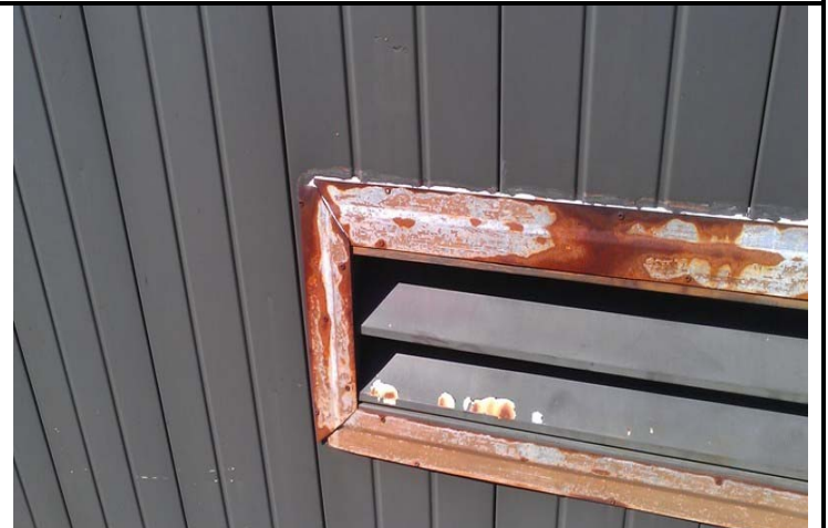
4. Built-up Roof #2 – View of White Caulk (ACM) along Vent, Samples # R43-44
