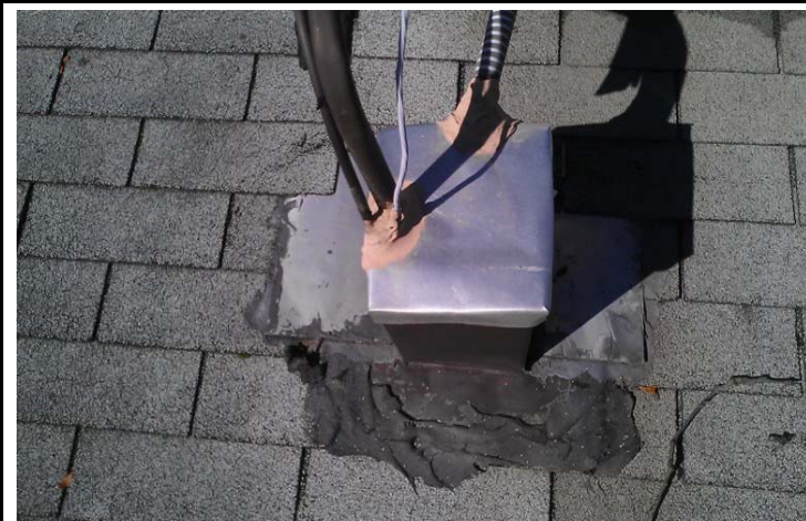
5. Built-up Roof #2 – View of Tar (ACM) By HVAC Unit, Samples # R45-R46
