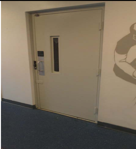
21. Assumed Asbestos-Containing Elevator Lift: Components. Not Sampled.
