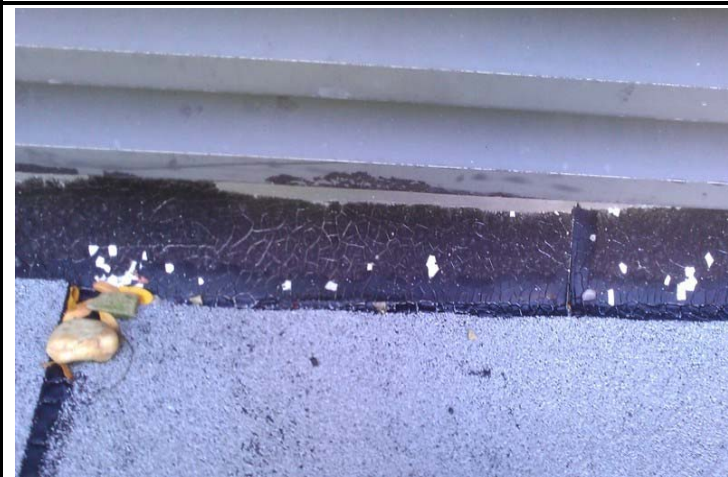
3. Roof of Lobby – View of Black Perimeter Flashing (ACM), Samples # R29-R30
