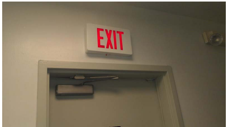
34. View of Exit Sign Assumed to Contain Lead-Acid Battery.
