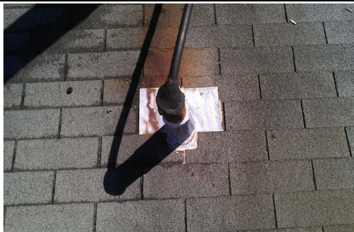
12. Built-up Roof #2 – View of Tar/Sealant on Electrical Supply Lines (Assumed ACM), Not Sampled Due to Safety Concerns
