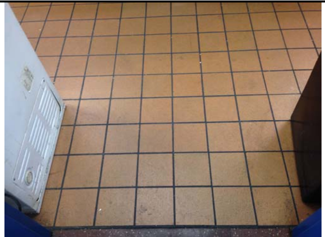
16. Assumed Asbestos-Containing Ceramic Floor Tile Mastic/Felt in the kitchen. Not Sampled.
