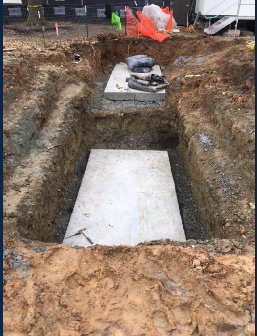
Concrete Pad for Splash Pad Vault
