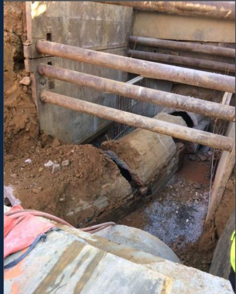
Removal Process of Existing Storm Line
