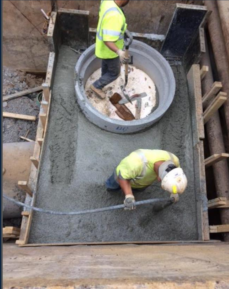
Cast In Place Manhole Structures for New Storm Line
