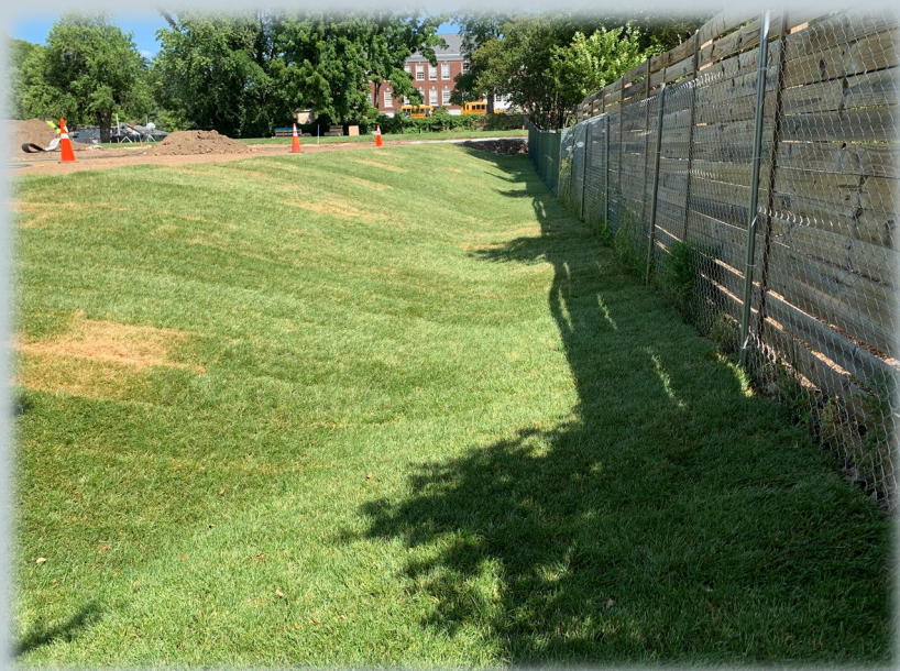
The sod has been installed below the lower field as well as in the swale.
