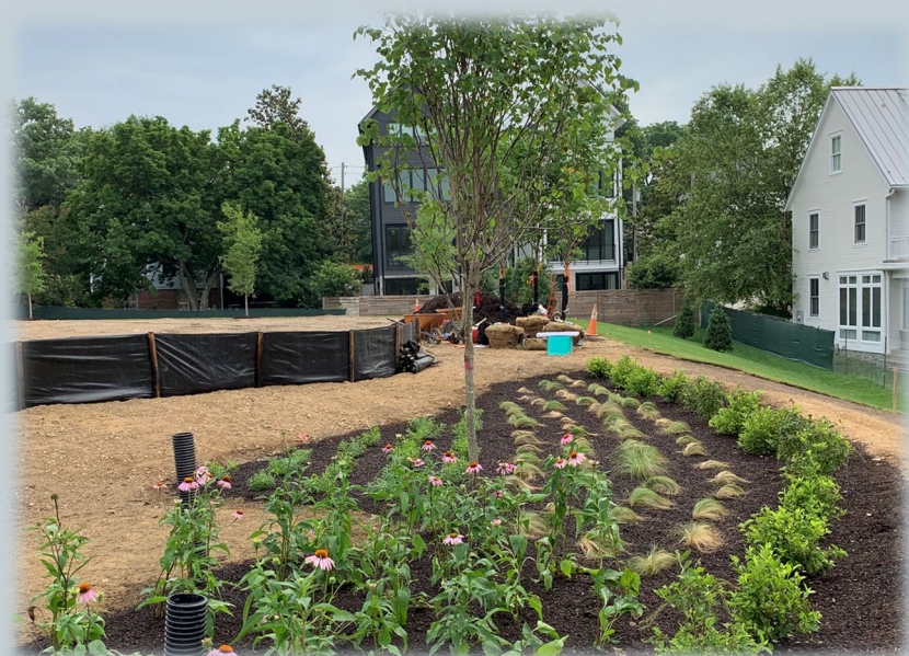
The trees and shrubs have been installed in the large field bio-retention facility.
