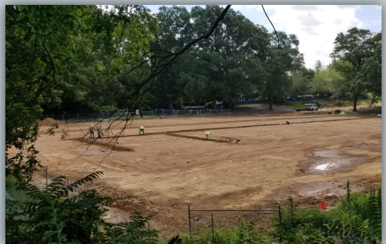
Field Irrigation being installed
