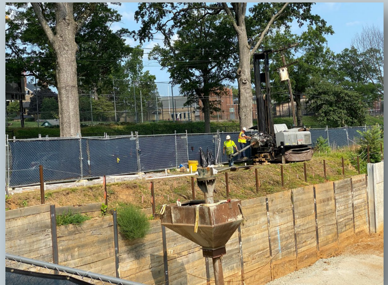
Well points being dug and installed
