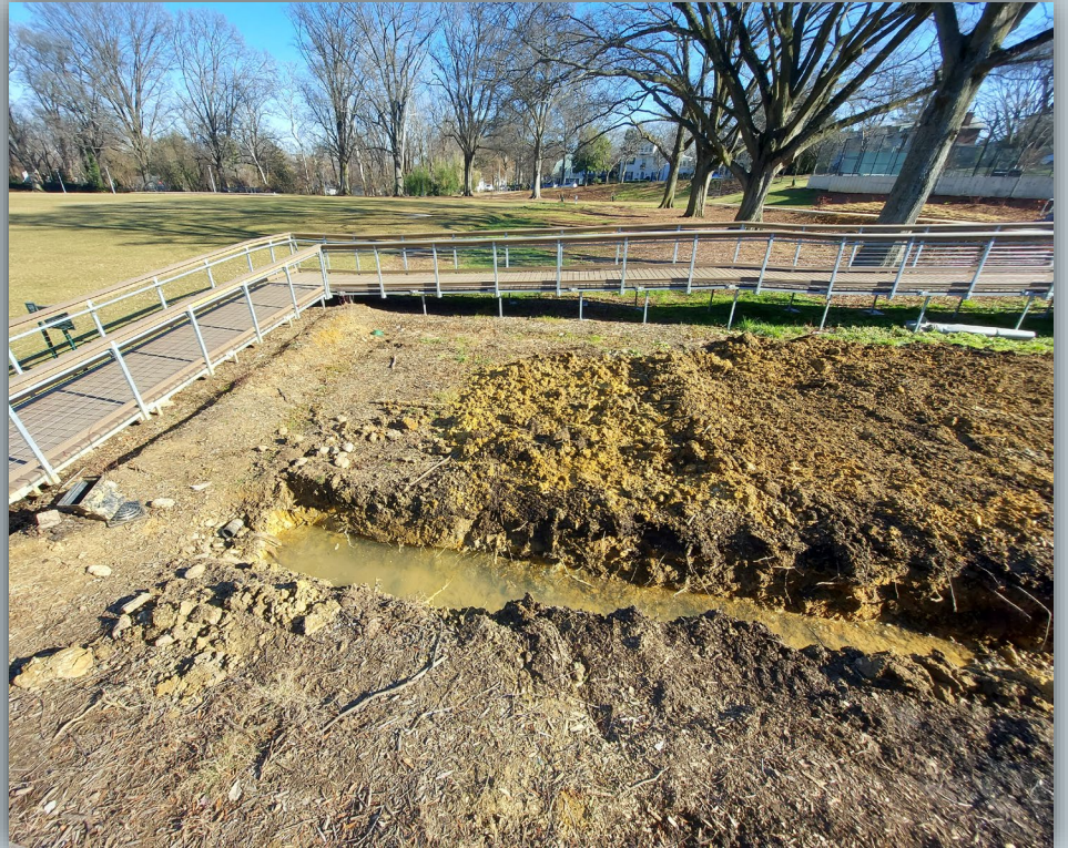
Water backed-up in the incomplete trench higher than the field as it flows down from the hill to the south to the field to the north.
