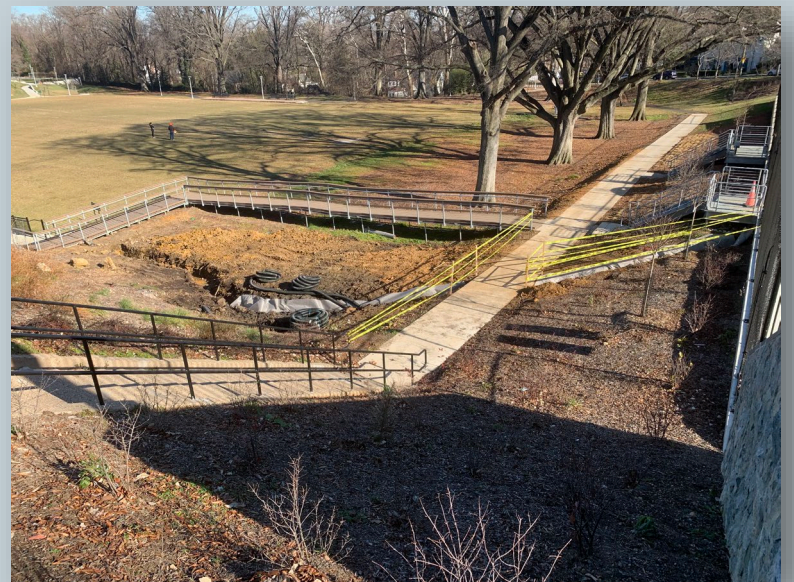
Trench has been dug for French drain.
