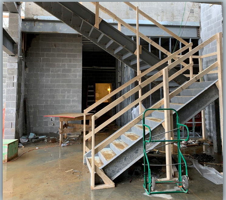
The Pool House stairs are now framed in steel
