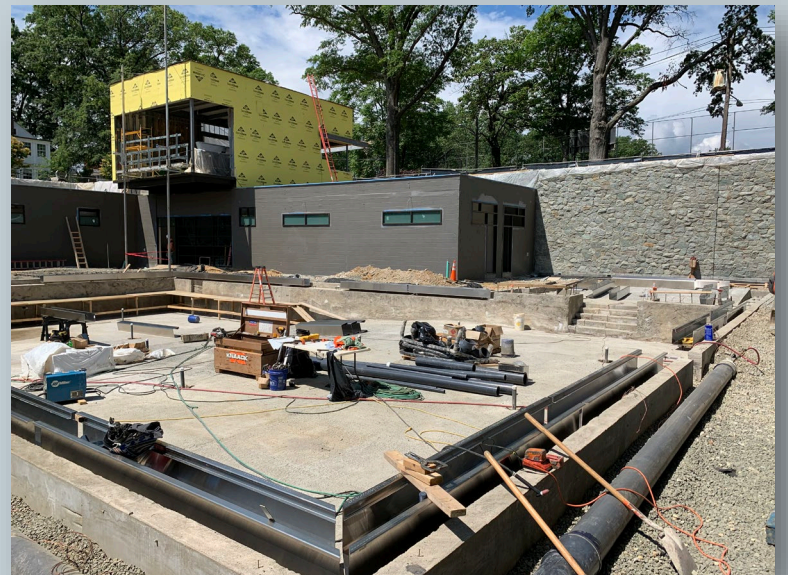
The pool concrete has now been poured and the pool edge is now being installed.
