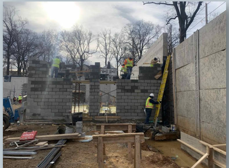
Masonry block Poolhouse walls being built
