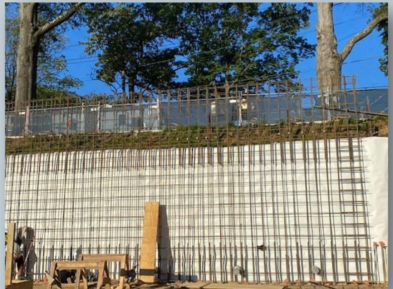
Rebar and Formwork for the building walls installed
