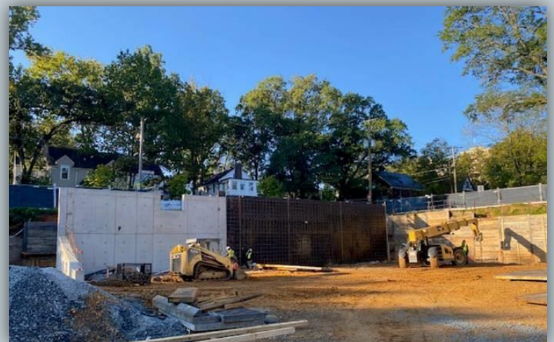
Waterproofing and concrete walls for the poolhouse
