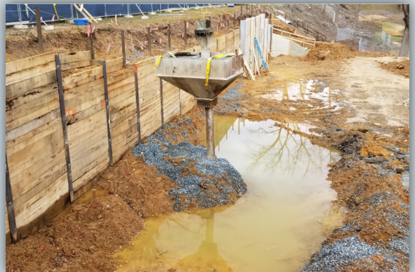
Water Intrusion into the work area causing water ponding
