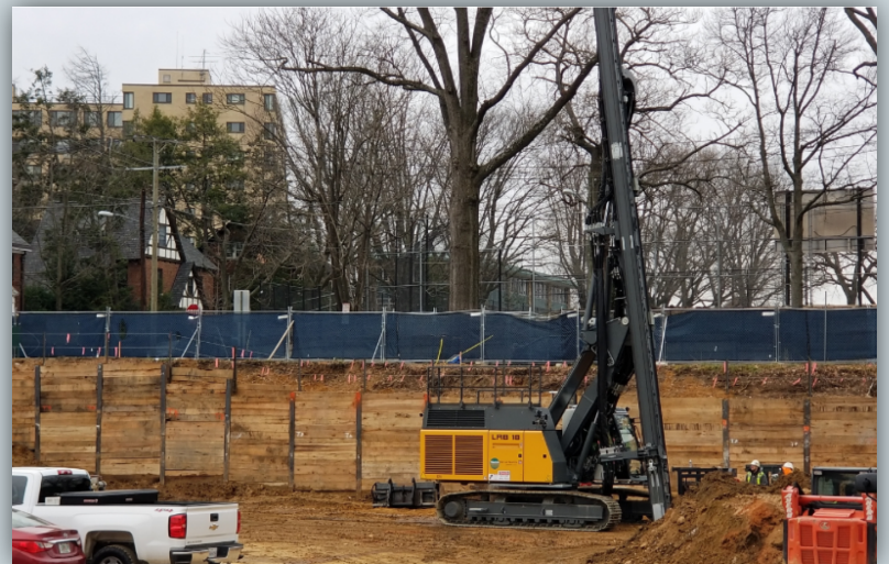
Piling and Drilling Rig installing geo-pier footings
