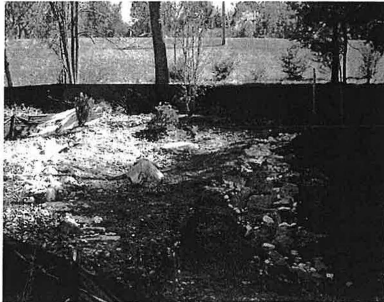
Figure 5: Step Pool Swale w/ Berms and Storage Pools
