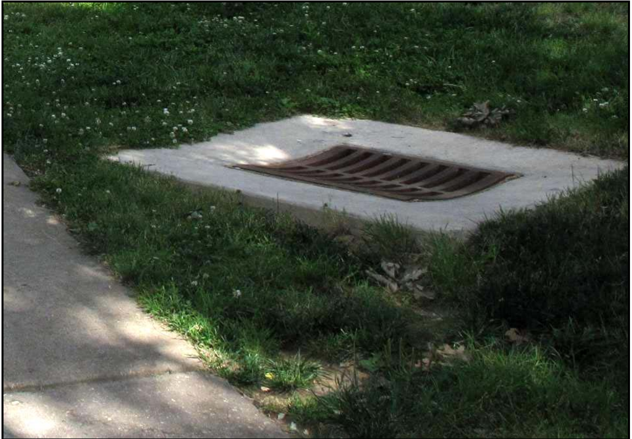
Catch Basin at Berm B3
