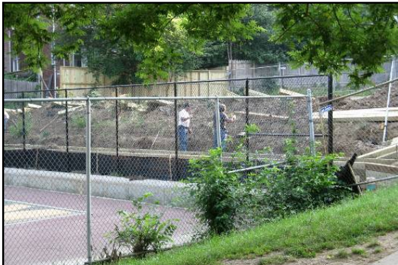
Photographs of construction of timber retaining wall.
