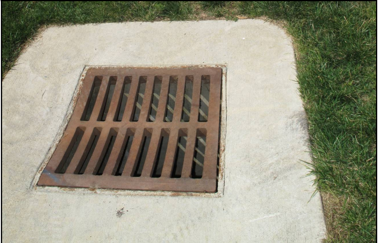
Catch Basin at Berm B2
