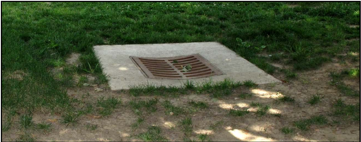
Catch Basin at Berm B1
