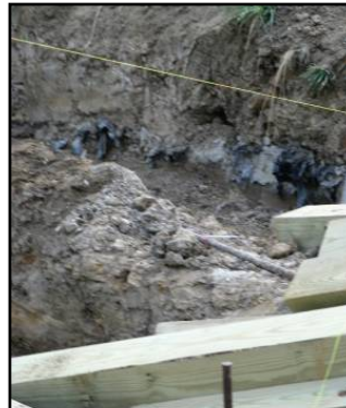
Photographs of construction of timber retaining wall.
