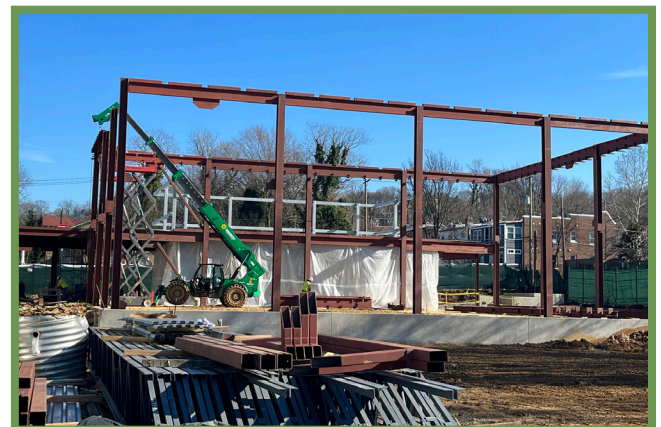
Exterior Framing for Gym
