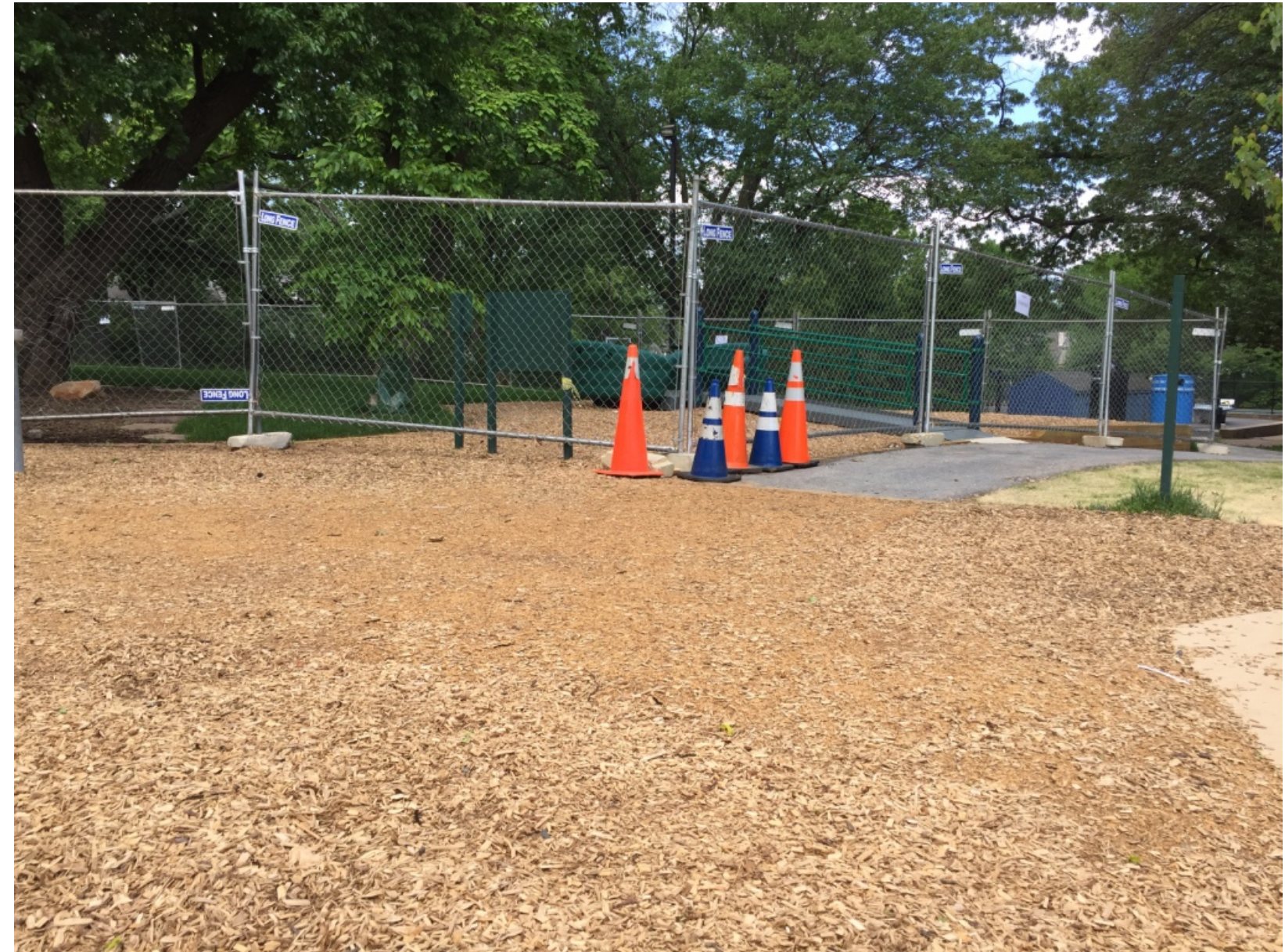
Installation of new surfacing and bonded wood carpet
