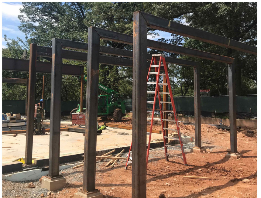
Structural steel installation.
