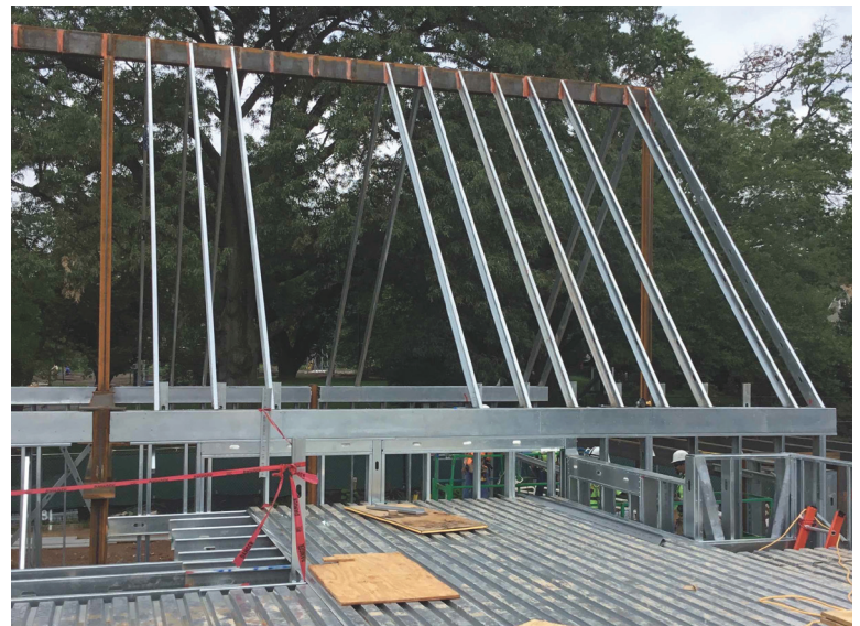
Roof frame and metal decking
