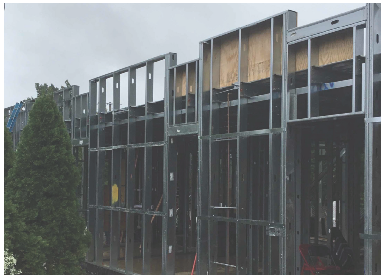
Structural columns and metal framing
