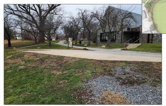
Removing the existing concrete pad and adding a bioretention area; borders to be built up Eco berms.
