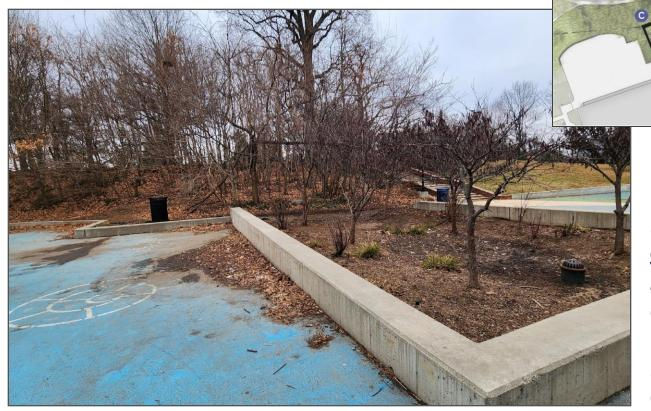
Existing bio: grading and new trench drain installation to stop sediment from coming over the wall.
