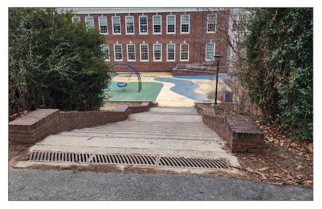
Existing conditions top of hill to the playground: the project plan is to modify the trench drain but remove stairs and shrubs and install a new retaining wall and bioretention area.
