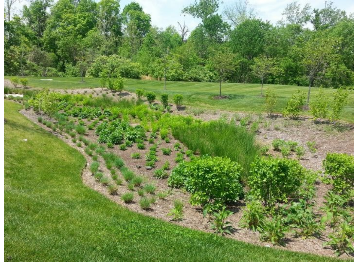
IMAGE OF BIORETENTION FACILITY
