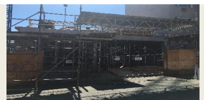
View From Clifton St. Parking Garage Structure Completion
