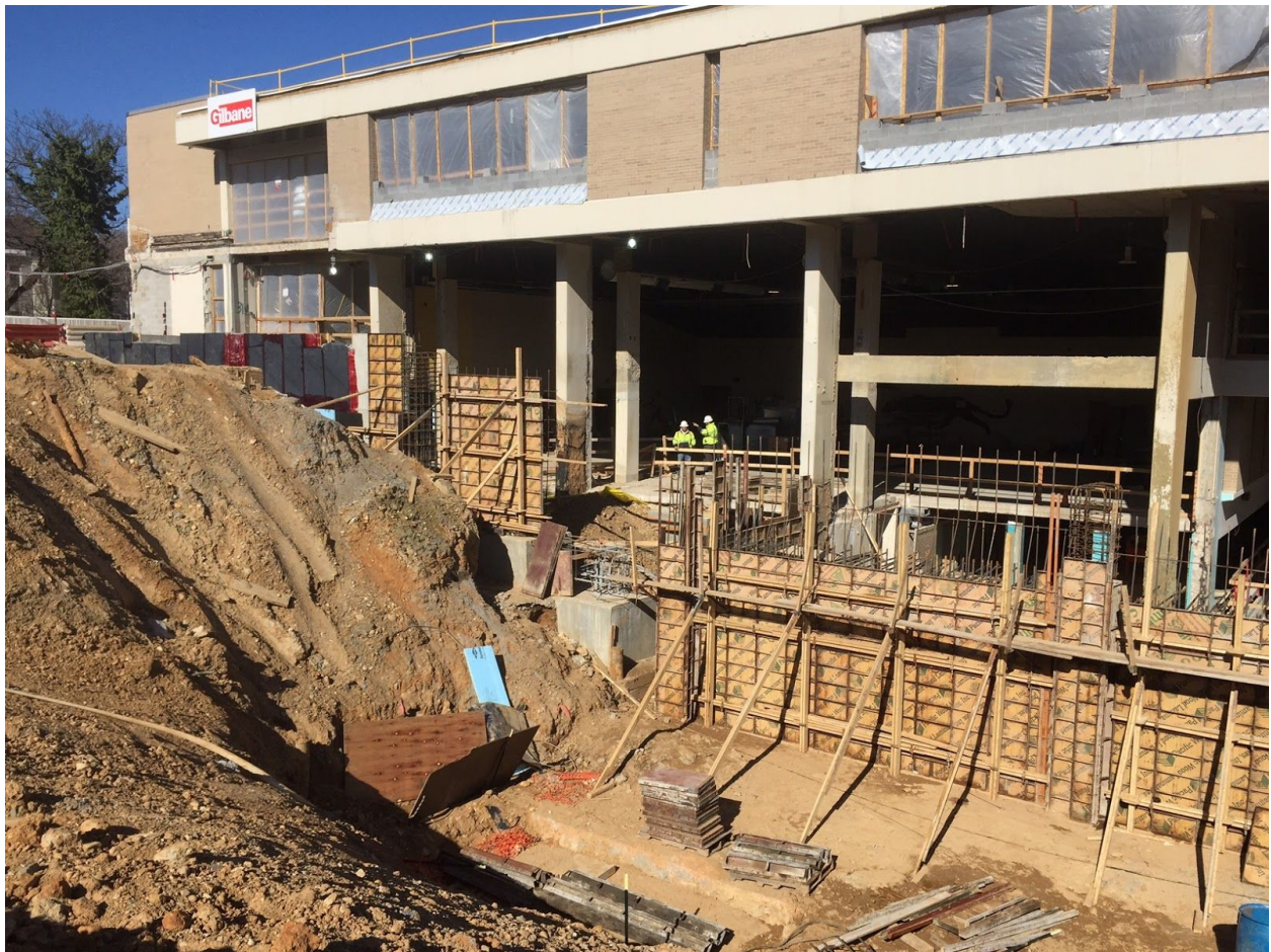
Concrete Formwork (at Main Entrance)
