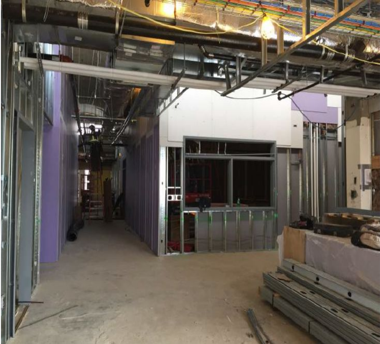
Gypsum Partition Work
