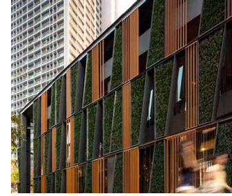
VERTICAL SHADING AT WEST FACADE
