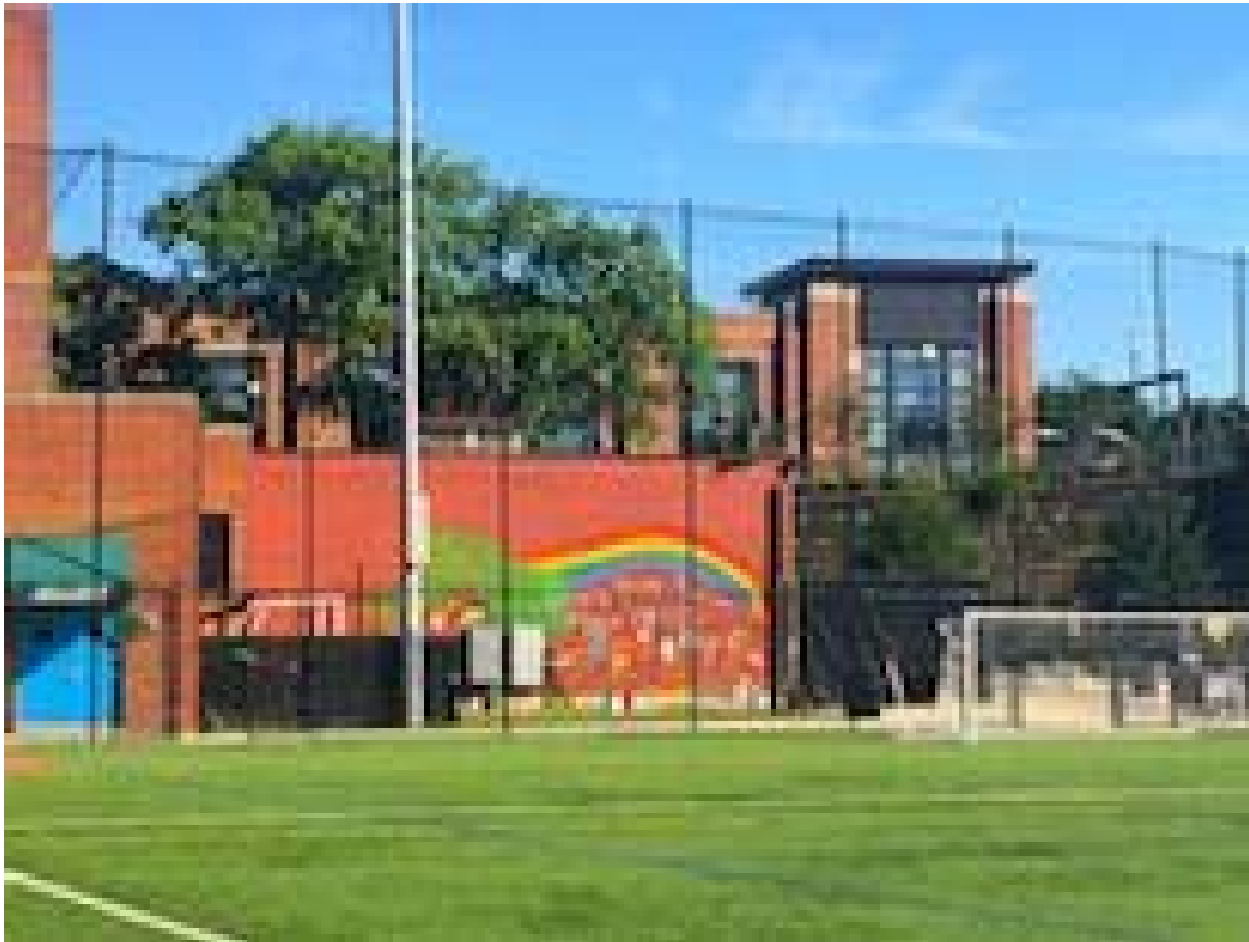
Image #1: Existing Structure
