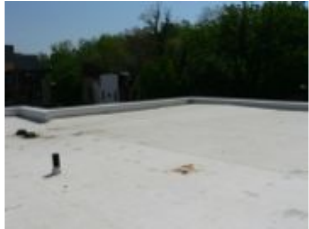
Figure 111: White membrane roof material on Sections 5-7
