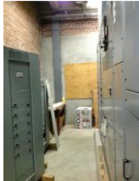
Figure 169: No space in the electrical room
