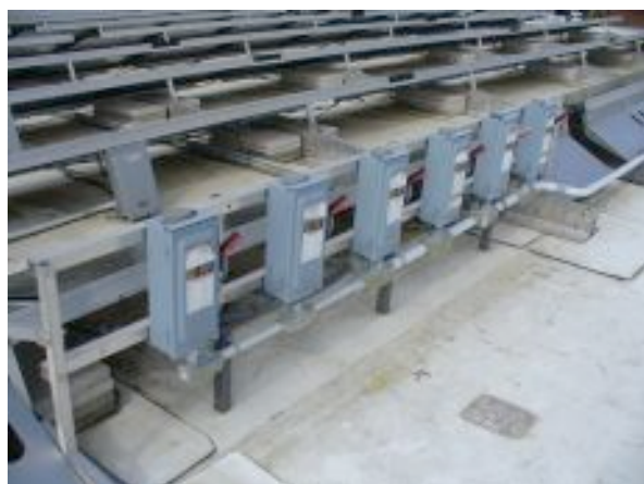
Figure 155: View of mounting system & DC disconnects
