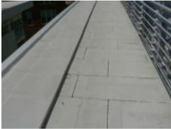
Figure 110: Ceramic tile roof material on Sections 1-4
