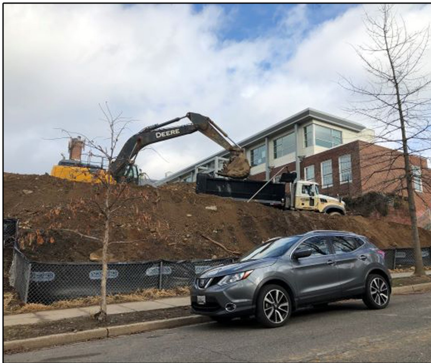
Excavation of soils in preparation for site sheeting and shoring.
