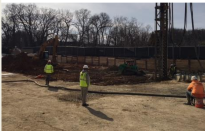
Auger Drilling Piles
