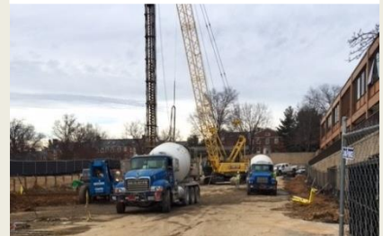
Grout Filling Piles
