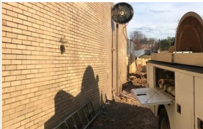
Retaining wall Demo
