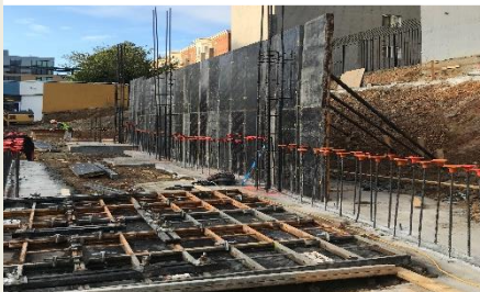
Site Retaining Wall Form Work
