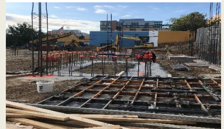
Concrete Column Rebar Work
