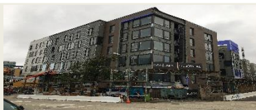
View of Façade Finishes from North-East corner of building.
