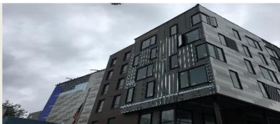
View of Façade Finishes from South-East corner of building.
