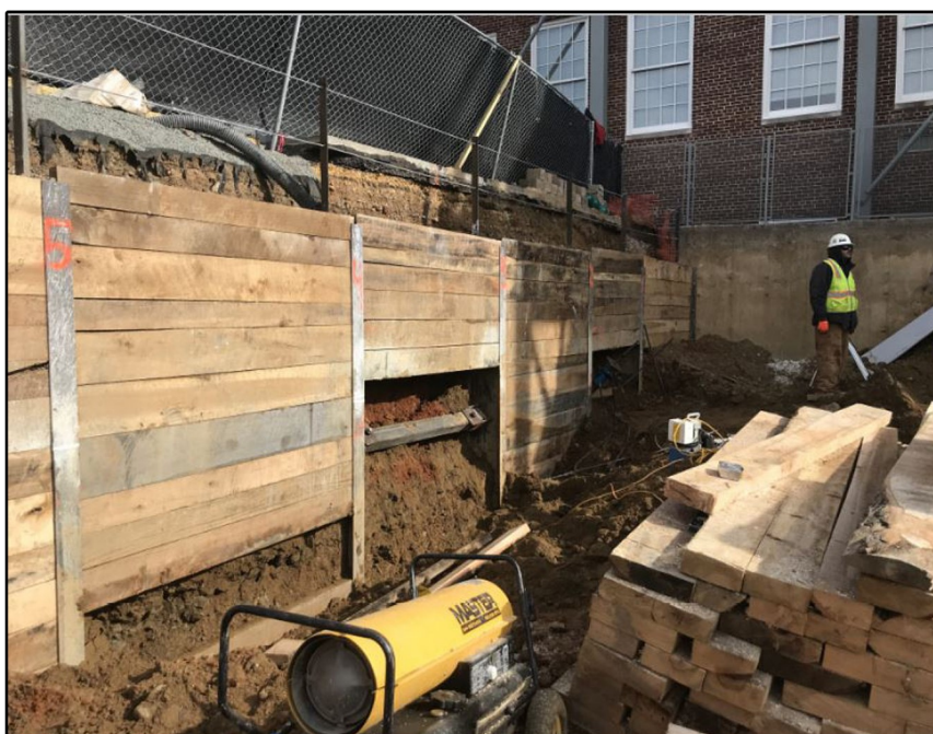
Soldier pile and lagging provides a temporary wall during excavation.
