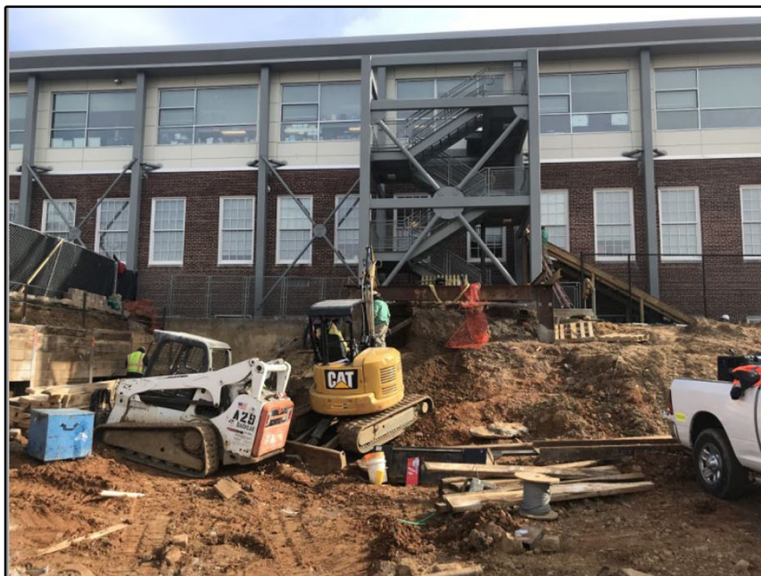
Excavation of excess soils in preparation for new addition.
