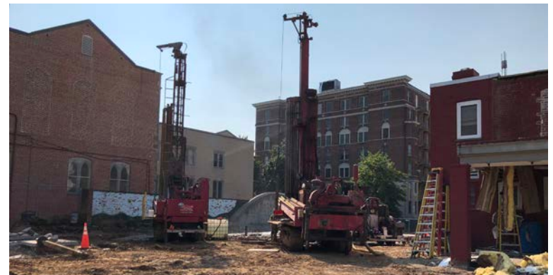
Geothermal well drilling
