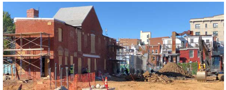
Site and carriage house addition demolition
