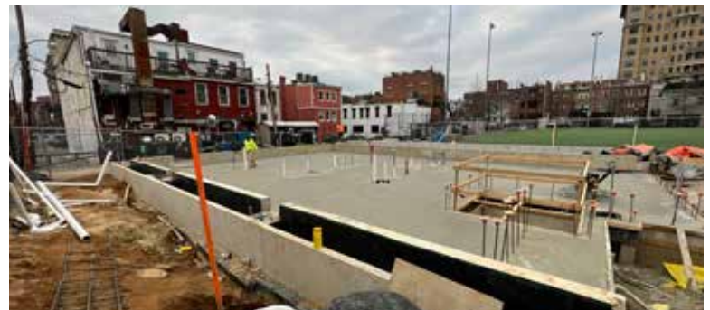
West slab-pouring - Under slab electric and plumbing
