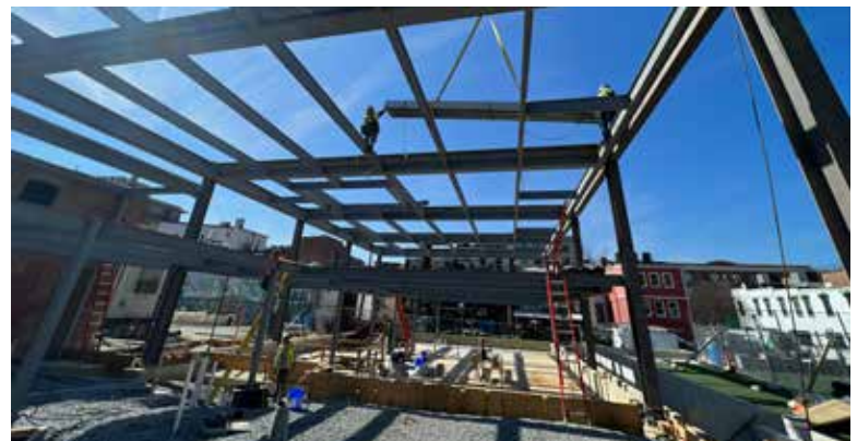
Structural Steel installation
