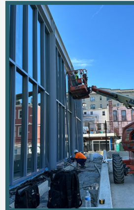
New building curtain wall installation.
