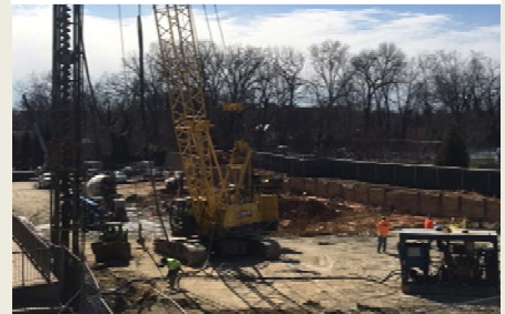
Grout Filling Piles
