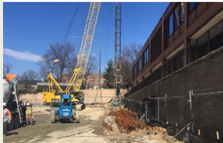
Drilling Auger Cast Pile
