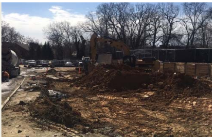
Demolition of Slab On Grade
