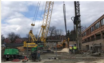
Auger Drilling Piles
