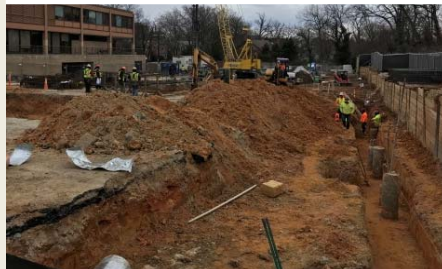
Excavation for Pile Caps
