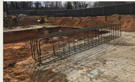
Grade beam Reinforcing
