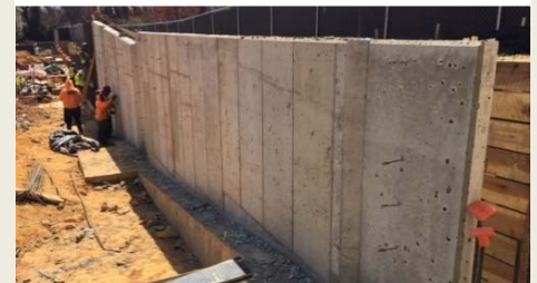
New retaining wall
