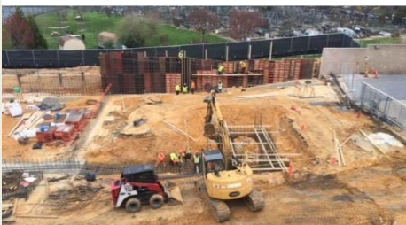
New retaining wall framing
