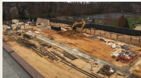
Grade beam pile caps
