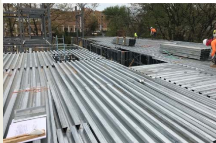
Metal Deck Installation
