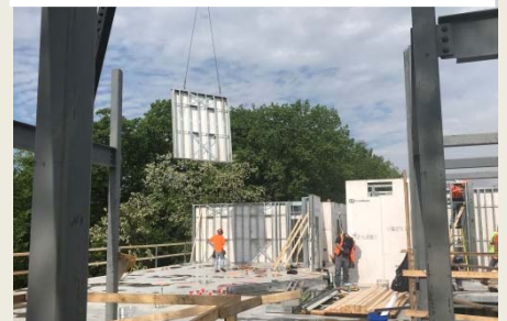
3 rd Fl. Structural Panel Install
