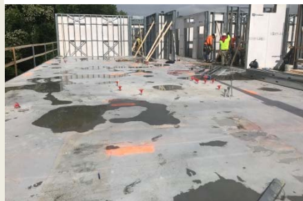
3 rd fl. Elevated Slab
