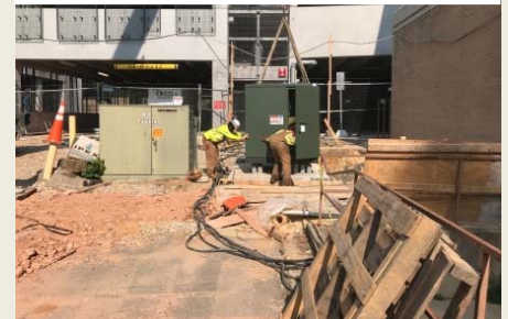
New Transformer installation
