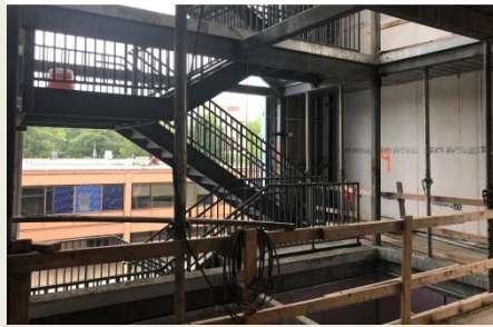
Metal Pan Stair installation
