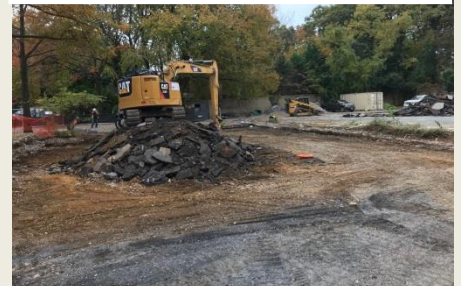
Asphalt removal - continued
