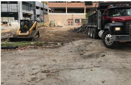
Asphalt removal
