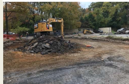
Asphalt removal - continued
