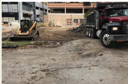
Asphalt removal
