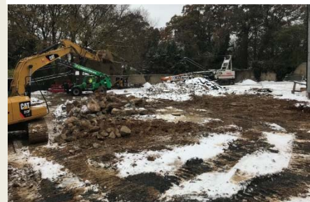
Asphalt & Concrete removal
