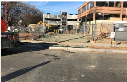
Second construction entrance
