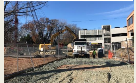
Debris removal in progress
