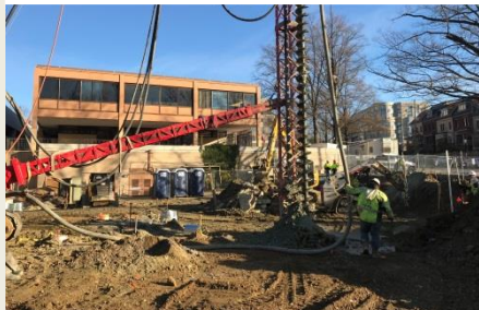
Drilling in progress
