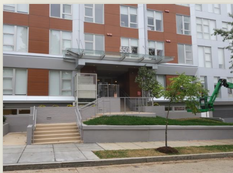
Completed Exterior Entrance.
